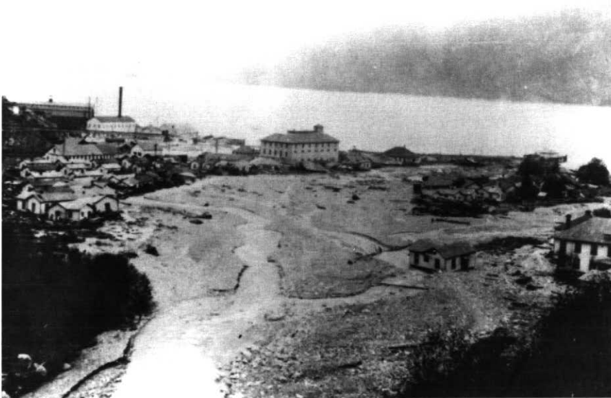
Figure 4b Telling the story with pictures: the mining community of Britannia, north of Vancouver, before (top) and after (bottom) the catastrophic flood of October 28, 1921 which killed 37 people (from Geoscape Vancouver ; Turner et al., 1996a).
