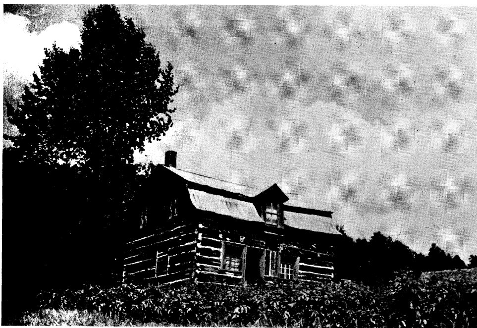
Photo 2 Square-timbered house near Lac Matilda, Harrington, with asymmetrical plan and gambrel roof.
