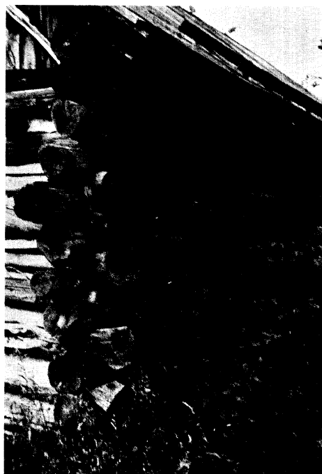
Photo 4 Saddle-notched cornering in a barn in Clyde Township, an area of French settlement.
