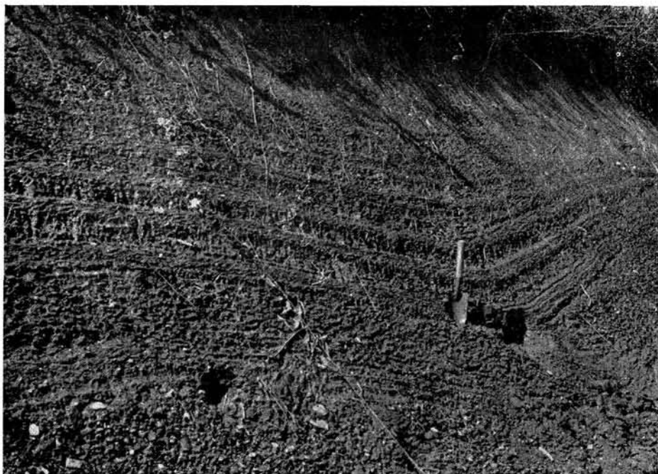
Small slumps in the lacustrine clays near Compton Station. The features are probably due to the melting-out of small ice lenses.
