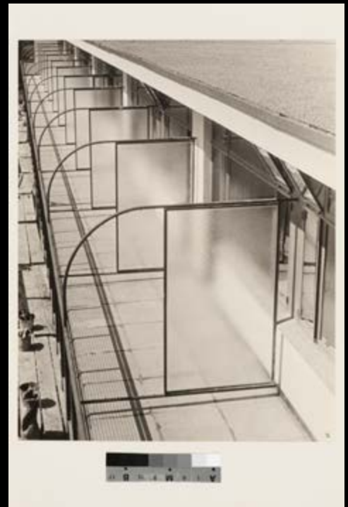
Ilse Bing , View of the glass partitions on the balconies of the Budge Foundation Old People's Home, Frankfurt am Main, Germany, 1930 , gelatin silver print / épreuve argentique à la gélatine, 28 x 22 cm, CCA Collection, courtesy of the / permission du CCA © Estate of / Succession Ilse Bing
